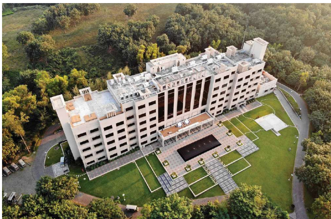
The Palace Luxury Resort – A project financed by Rupali Bank Limited
